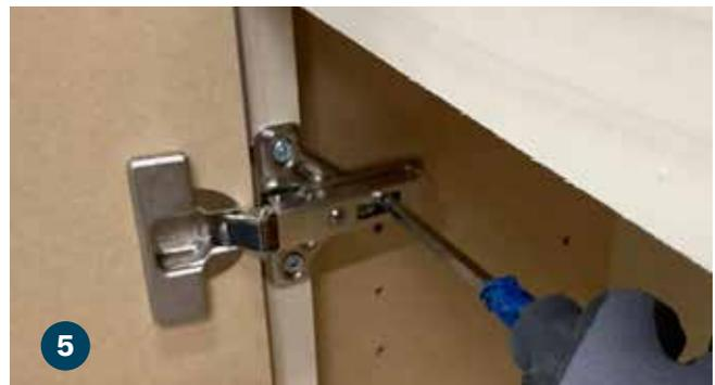
Use the screws in the hinge to adjust door placement. The front screw brings the door to and from the center when the cabinet door is closed.
