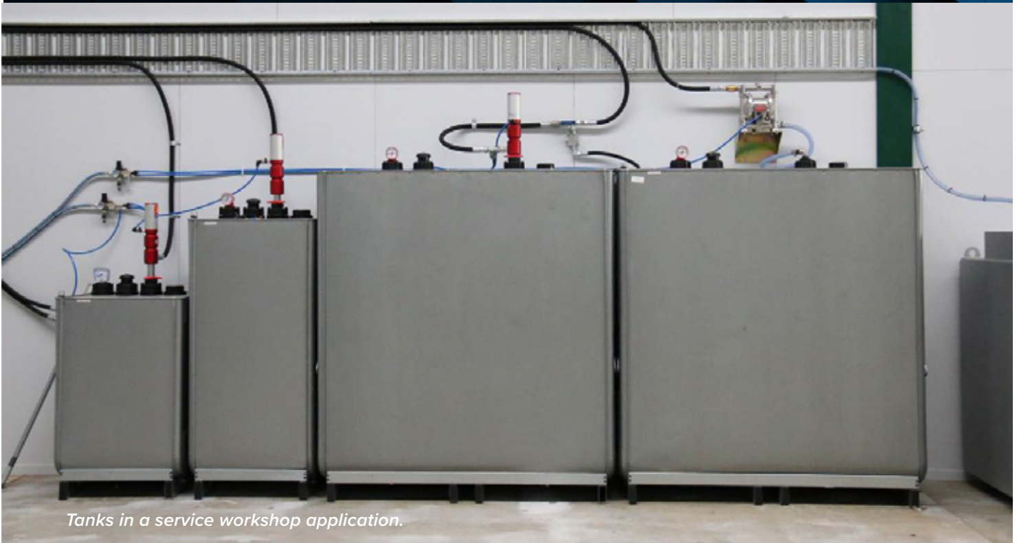
Self-contained tank setup with top mounted reel and drip tray / gun holder.
