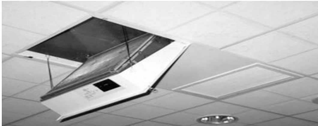
Easy access filter cell/HEPA filter in drop-down door.
