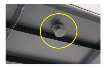
8. Install the four provided Plastic Rivets in the holes drilled in previous step to complete installation.
