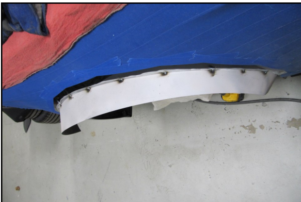
21. Continue to place tack welds in alternating locations along the extensions inner and outer edges as shown.
