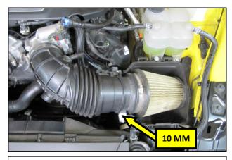
**9.** Using a 10 mm socket, remove the bolt securing the intake tube and filter to the lower half of the air box.
