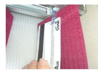
**4.** Remove the louver by pulling down on both the louver and the plastic card at the same time. Lay the louver on a clean, flat surface. Repeat for all louvers.
