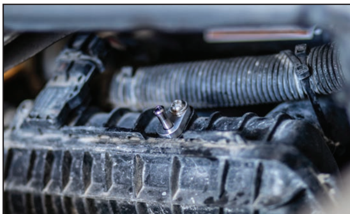
PORT FITTING INSTALLED
