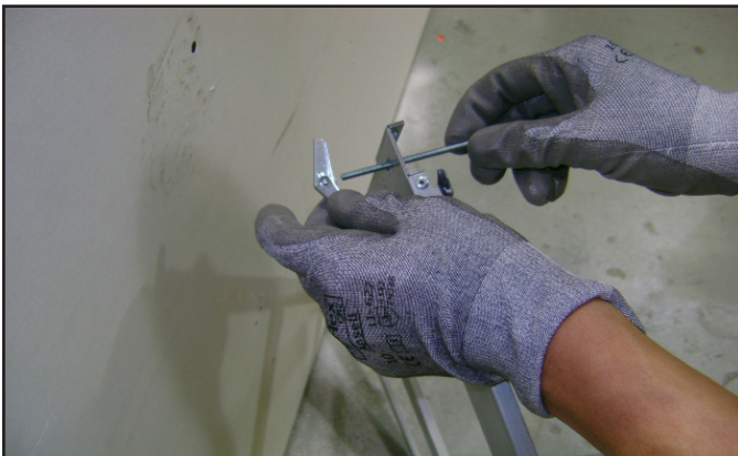
Figure 4.5 Toggle Bolt Installation through Mounting Bracket
