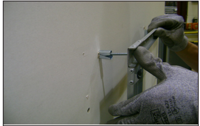
Figure 4.6 Installing Anchors in Hollow Wall
