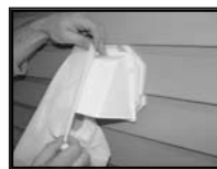
Position LintCatcher over the vent
