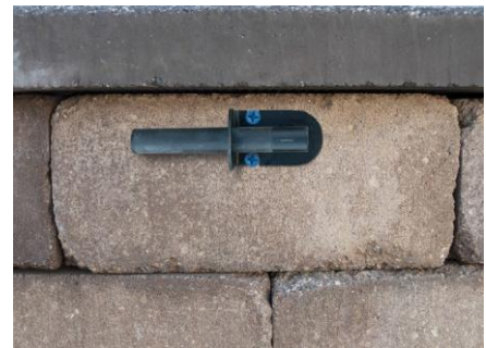
Figure 6.6 – Fasten down the bracket
