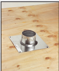
Push pipe through vent support.
