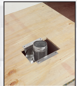
Push pipe through vent support.
