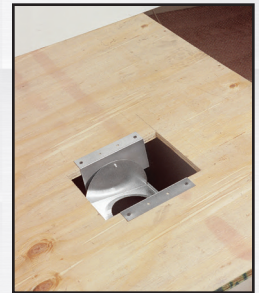
Mount SureGrip support plate.
