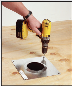
Mount SureGrip support plate.
