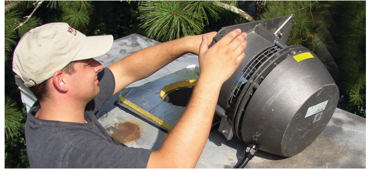
Installing the fan on top of the chimney is fast and easy.
