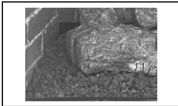
Figure 44 - Installing the volcanic stone
