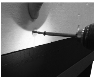
Step 3: Top of front fireboard standoff should be flush with top standoffs (not shown).
