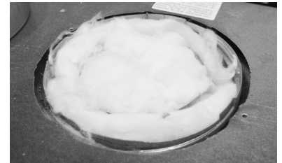
Step 3: Remove insulation from inside flue pipe.
