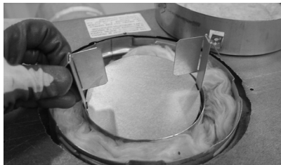
Step 4: Make sure insulation disc is still in the round cover. Remove the flue plug from the top flue.
