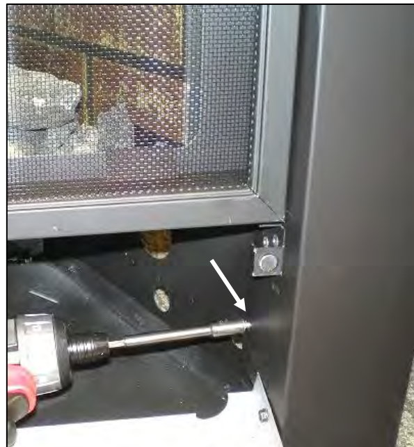
Step 4: Open Lower Panel and install screws through surround. Raise Lower Panel and replace screws.
