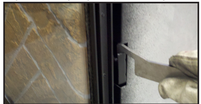
Figure 11.7. Securing Side Glass Clips
