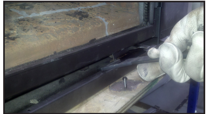
Figure 11.2. Glass Clip Tool Location
