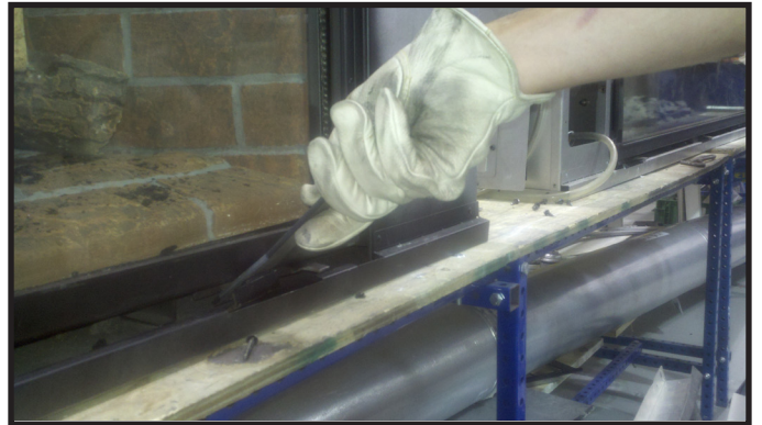
Figure 11.3. Inserting Glass Clip Tool
