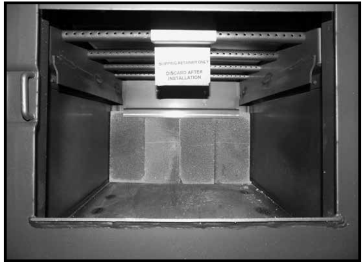
Figure 20: Bricks against rear wall.
