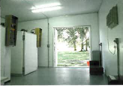
Emu Incubation Chambers require that a constant internal temperature be maintained. The continuous insulation and high thermal rating of the 8" Snap-N-Lock Insulated Panel made it the perfect choice for this application (both the interior and exterior view shown).
