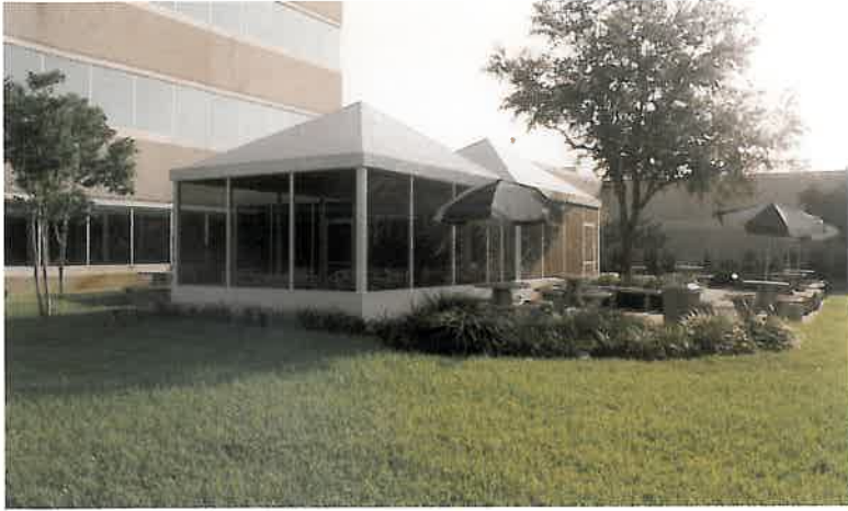
The attractive roof angles of this outdoor covered lunch area were constructed of Snap-N-Lock Insulated Panels.
