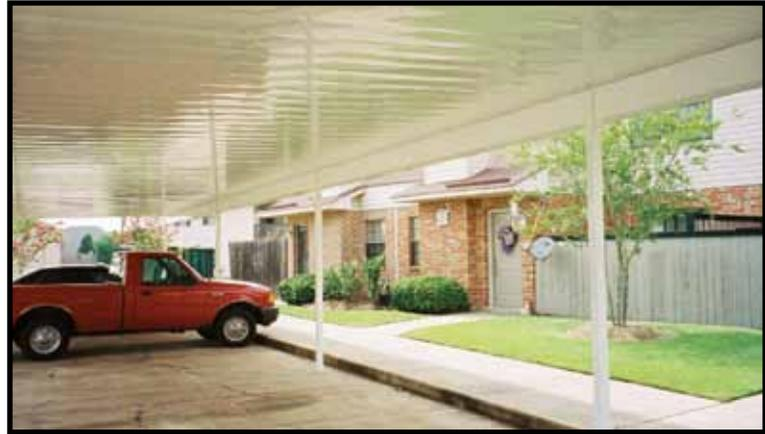
*Below: This gabled walkcover constructed of roll-formed pan is structurally more sound, drains better, and offers an aesthetically interesting walkcover.*
