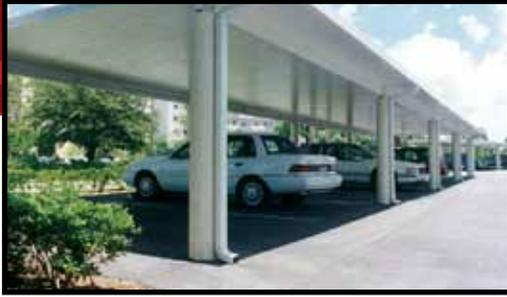
*Below: Snap-N-Lock Panels™ can span large distances with less support than other building materials, as you can see in this Florida school walkcover.*
