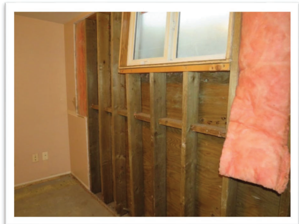
Fig. 1-17 Bowed PWF Wall
