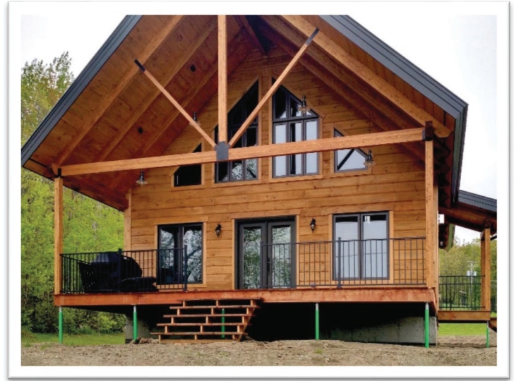
Fig. 1-20 Green Helical Piers Supporting Deck
