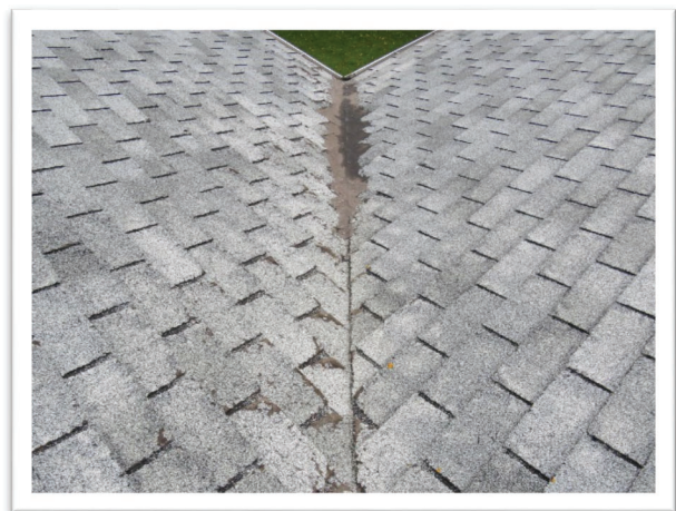
Image 7-7 Lower Valley Deterioration
