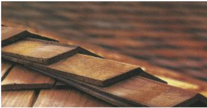
Fig. 7-8 Cedar Shingle Hip Capping
