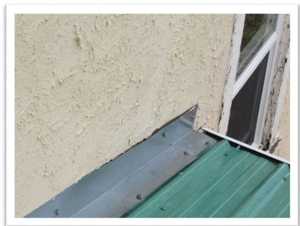
Fig. 7-14 Improper Wall Flashing Installation
