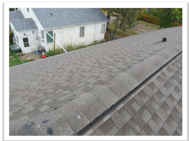
Fig. 7-10 Shingled Continuous Plastic Ridge Vent
