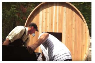
To install the wood burning heater, lift the heater into the hole in the back of the sauna.
