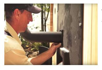
Attach the chimney elbow to the wood burning stove by pushing the provided bolts into place and hand tightening the nuts on the other side.
