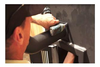
Using a wrench to hold the nut on the inside, tighten the bolts completely with an impact drill or a wrench.
