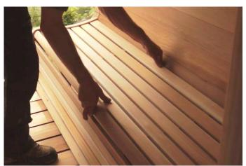
Place the bench seat on top of the installed front assembly as shown.
