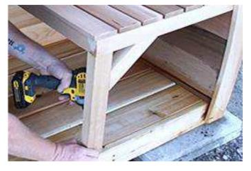
Screw the outer leg of the assembly to the floor using a 2 ½" Kreg screw in the pre drilled hole.
