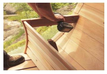
Join the bench supports at the top of the bench front by their square ends with two kreg screws. Level the Bench Support, and join the angled end to the sauna wall with two Kreg screws, as shown.
