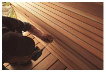
Secure the top of the bench to the bottom assembly in the front with two 2½" deck screws (2 places, as shown below)
