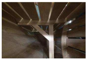
Before fastening top bench to front assembly, Screw bench bracket to bench support using 2" screws.
