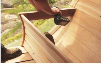
The sauna interior benches have a support at each end and supports in the middle of benches.
