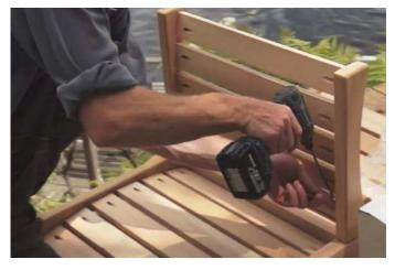
Assemble porch benches (if applicable) by fastening seat assemblies to front assemblies using one 1½" Kreg Screw per joint (2 joints)
