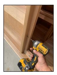
If your sauna door is twisted or crooked loosen the screws from the top and bottom of the door so you can straight the frame and re tighten the screws. It is recommended to remove the door from the frame and do this with the door laying down on a flat surface. We also recommend re-positioning the screws so they do not end up in the same hole pattern as before. Wood glue should be applied. Photo Below.
