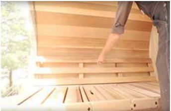
Install backrest with 2" screws at desired height making sure that the lounge bench can still operate correctly.
