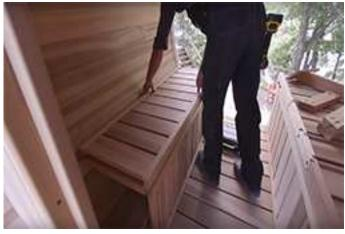
Ensure bench is flush and secure with 2  $\frac{1}{2}$ " screws.
