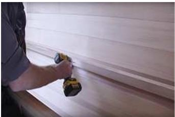
Position assembly in place and secure to sauna walls and floor using 2  $\frac{1}{2}$ " screws.
