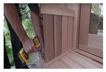
Fasten bench to floor and sauna wall using 2  $\frac{1}{2}$ " screws.
