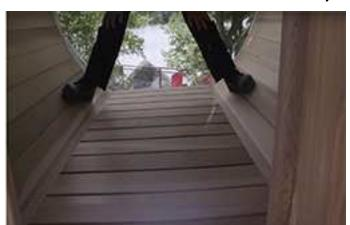
Install the flat floor in the middle of the sauna making sure it is level.
