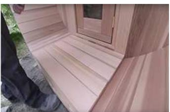
If the porch option is selected, start by installing floor ensuring it is level.
