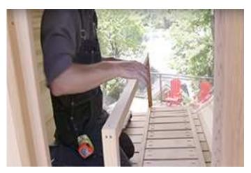
Using the pre drilled holes, assemble the lounge bench support to the longer front lower bench wall using 2" screws.
