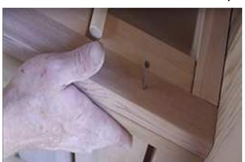
Ensure bench is flush with bench support and secure with 2 ½" screws in pre drilled holes.
