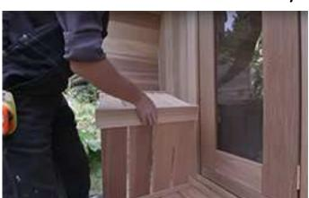
Assemble the 2 pieces for the porch seat together using 2  $\frac{1}{2}$ " screws.
