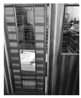
3. Take the front large panel with glass door and place on base. Be careful to not allow the door to swing and accidentaly break the glass.
