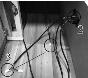
4. Lay the second bench down half way and connect the heater cable labeled "4".
