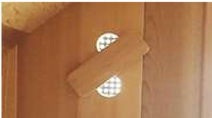
Install the cedar vent cover over the outlet holes on the inside of the sauna with a 1 ½" screw.
