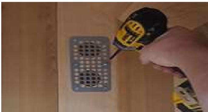
Install the other Stainless Vent cover over the outlet holes on the outside using 1-1/2" stainless steel screws. (6pcs)
