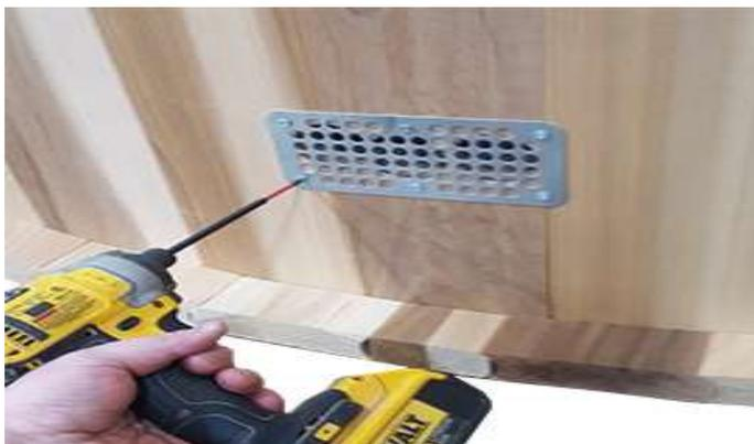
Install 1 of the stainless steel vent grills over the inlet holes on the outside of the sauna centered over the holes using 1 ½" screws. (6pcs)
