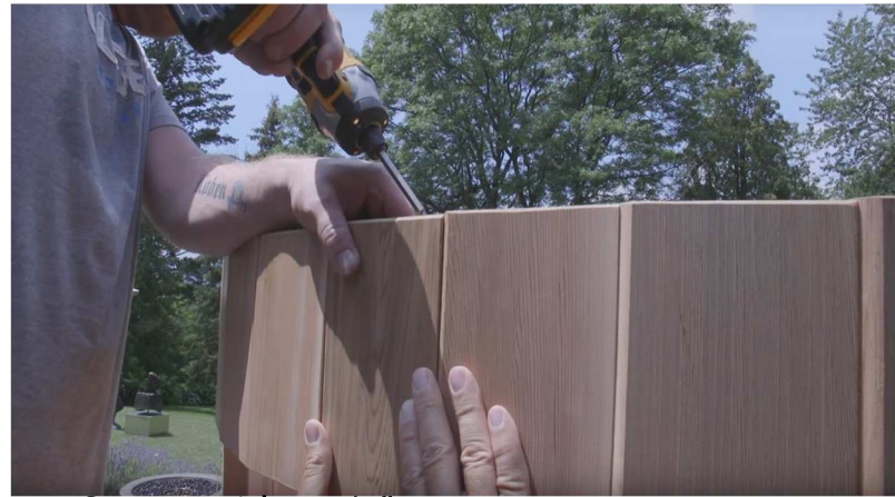
20. Secure with 2 1/2" screws.
