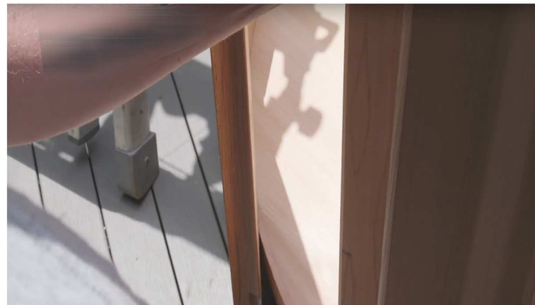
17. Carefully angle out the 2 adjacent staves and insert the double stave.
