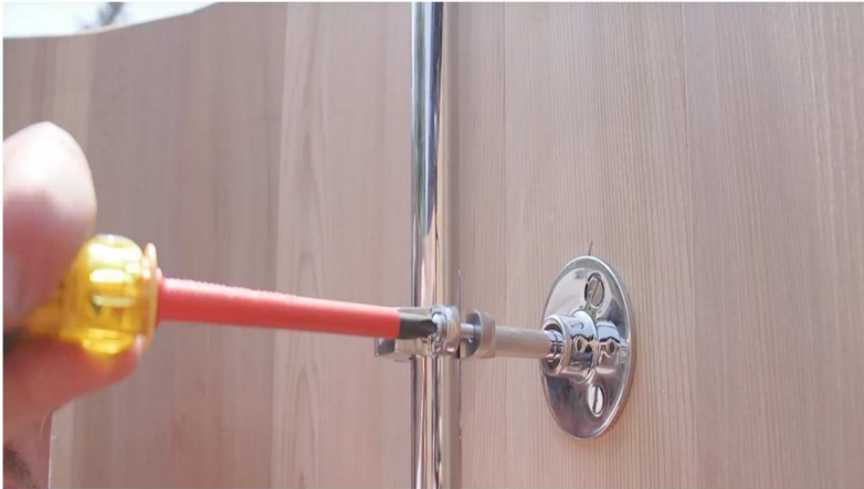
36. Tighten support snugly ensuring shower head faces forward.
