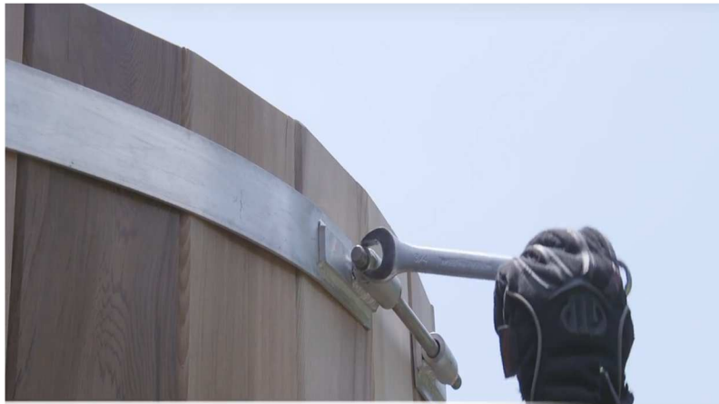
30. Use a wrench to ensure both bands are very tight. Hearing the wood creak is common.
