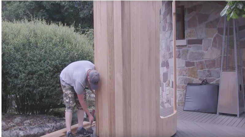
14. Use rubber mallet if required.
