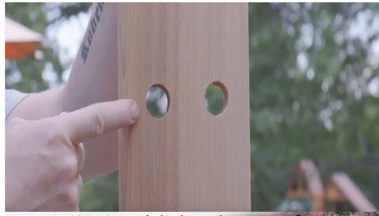
15. Insert Stave with holes adjacent to floor drain. Continue attaching staves.
