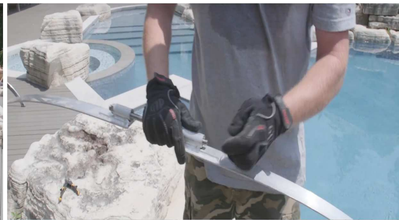
22. Bring the ends together of the first band and connect them using the provided threaded rod and nuts as shown.
