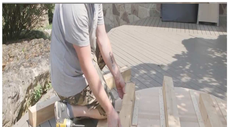
6. Place wood supports across the floor pieces, longer pieces on inside, shorter pieces on outside. Ensure wood supports are centered and not covering the outside bessel.
