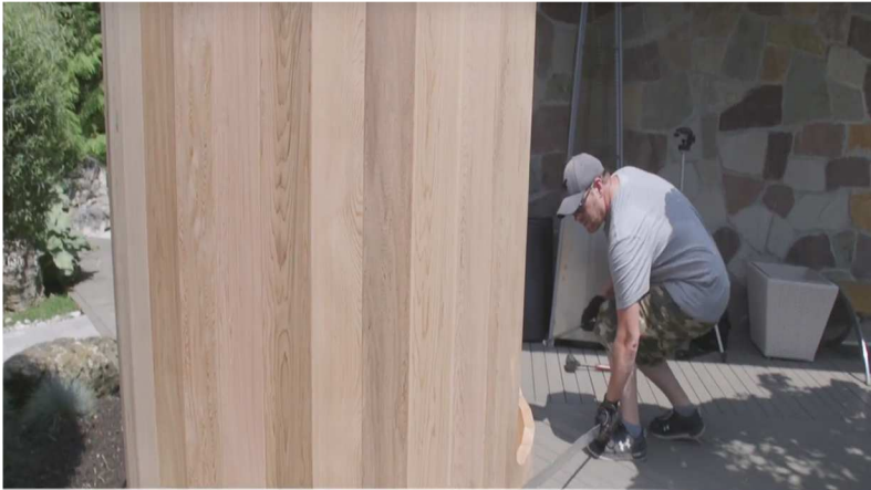
25. With a helper, wrap the second band around the bottom of the shower and connect the ends in the same manner as the top band.
