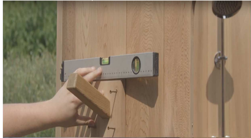
37. Attach towel hanger in your preferred location using 1 3/4" screws.
