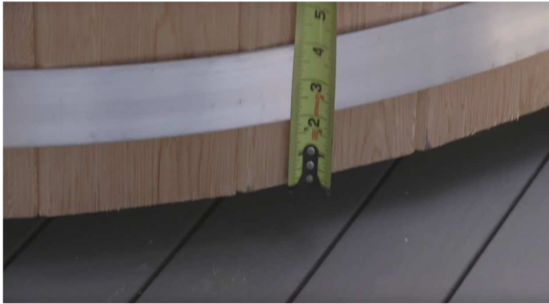
25. With a helper, wrap the second band around the bottom of the shower and connect the ends in the same manner as the top band.
