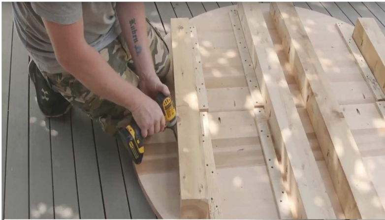
7. Secure wood supports with 2 1/2" screws.
