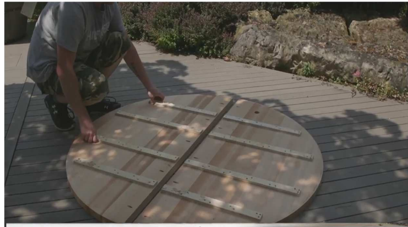
2. Start by placing both floor pieces on level ground.
