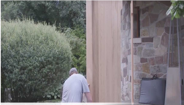
13. Continue adding staves clockwise around shower ensuring staves are tight together.
