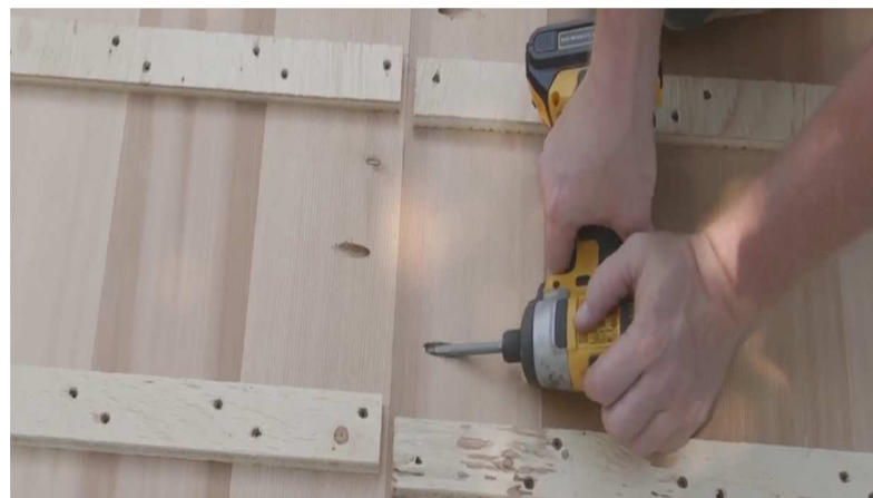
5. Screw together using 2 1/2" screws.
