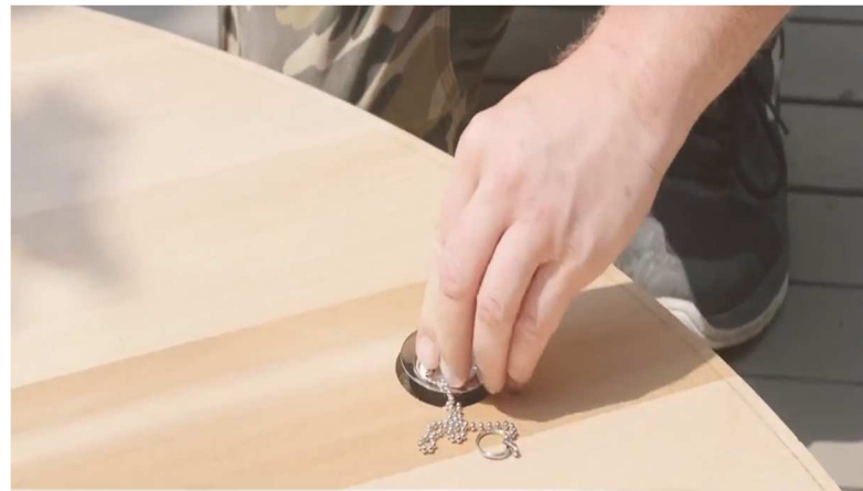
9. Insert drain into hole in floor, tighten firmly.
