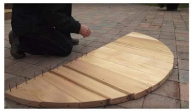
Line up cove pieces starting with smallest pieces on ends and working towards the middle forming a semi circle. Place 2 1/2" screws in predrilled holes to assist in assembly of cove.
