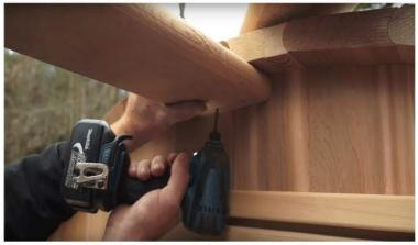
Secure with 2 1/2" screws from underneath
