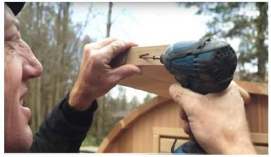
Screw 2 1/2" scews into pre drilled holes on end to secure cove pieces together.
