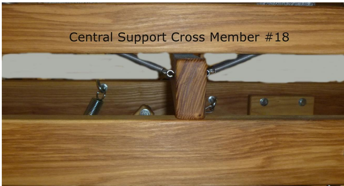
Figure 22 - Central Support Cross Member
