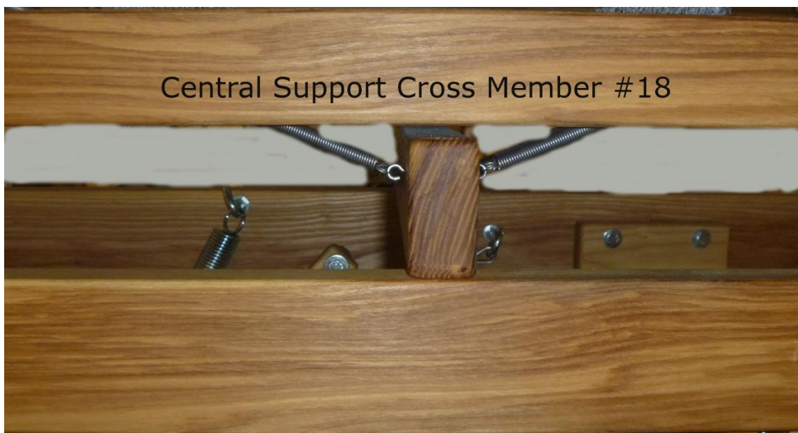
Figure 22 - Central Support Cross Member
