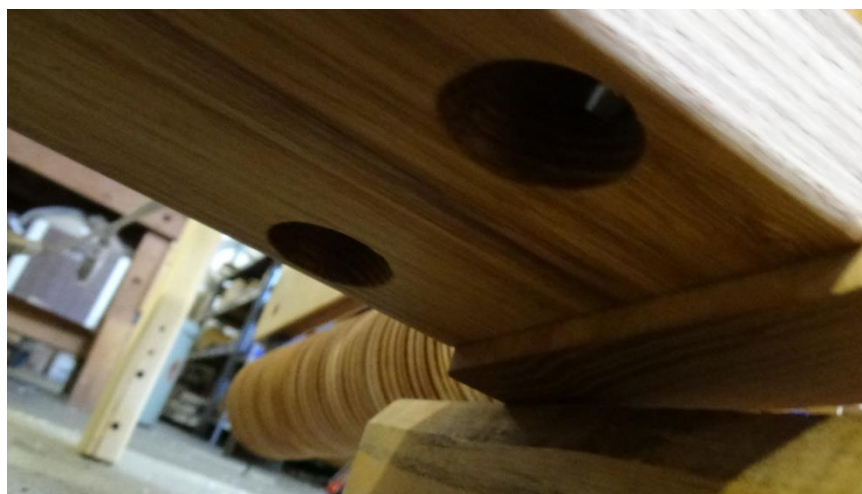
Figure 18 – Closeup of nut access holes
