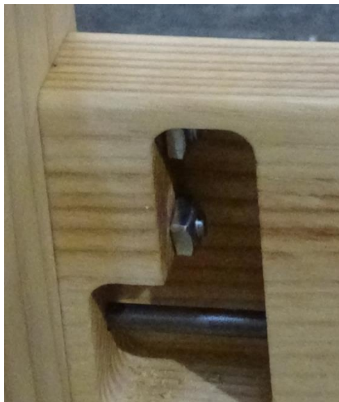
Figure 15 - Front cross member attached to side frame
