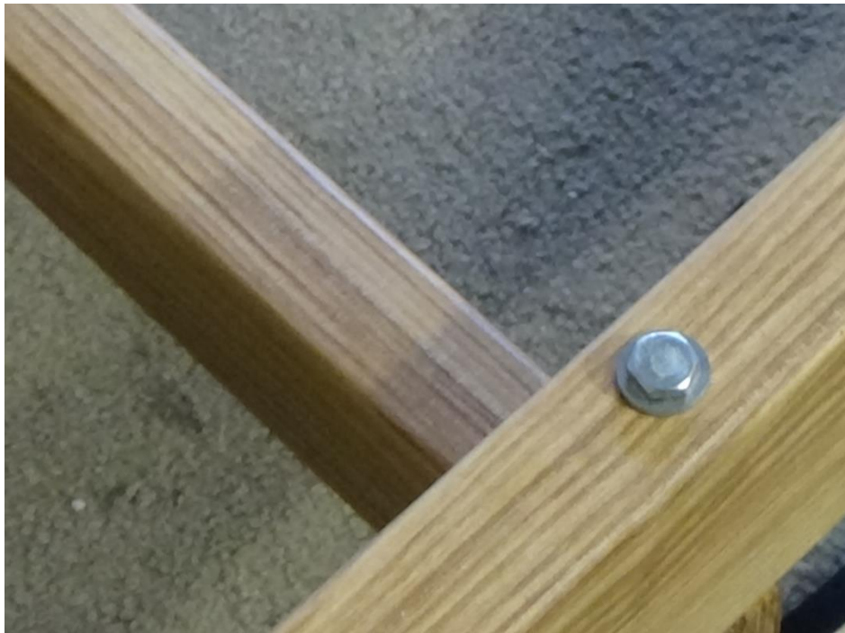
Figure 13 – Bolt for bottom harness pulley support assembly
