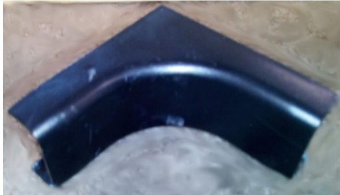
Figure 9 - Connection cover
