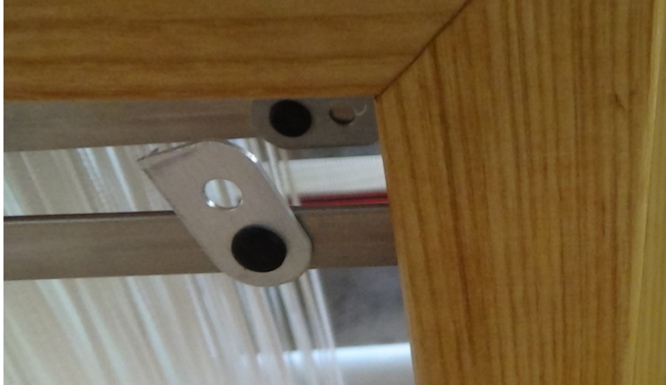
Figure 35 - Keeper on harness opened from back
