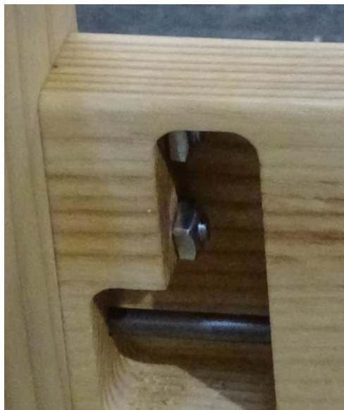
Figure 15 - Front cross member attached to side frame
