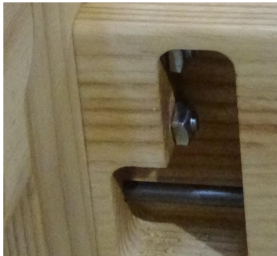
Figure 48 - Beater support pins
