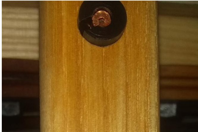
Figure 9 - Nico secured with cable button
