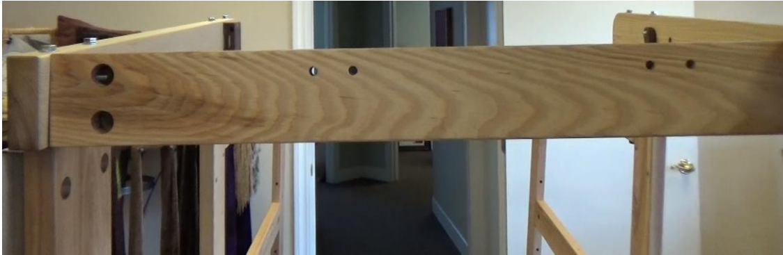
Figure 25 - Attaching front crossmember
