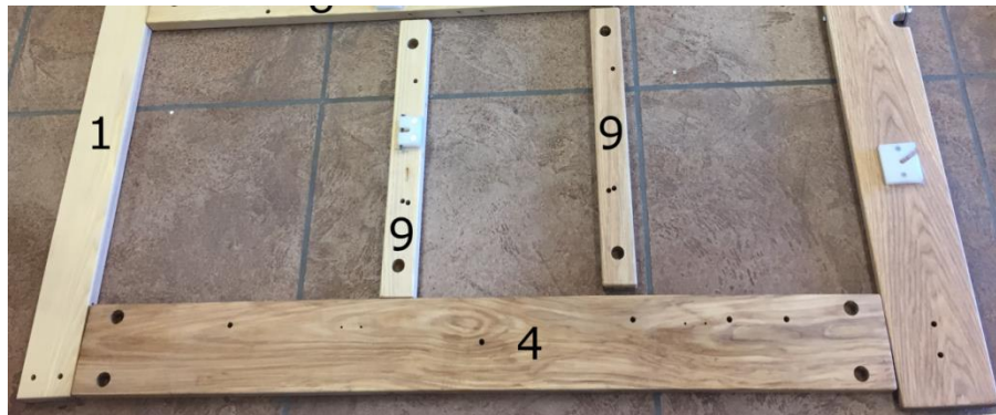
Figure 17 – Partially completed side frame
