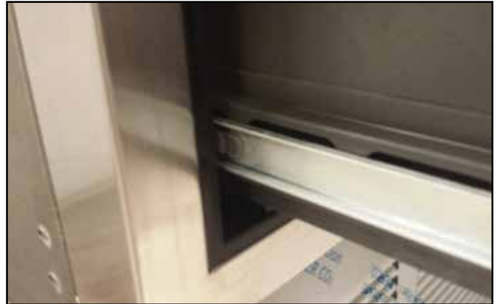
Figure 8-15.1 - Freezer Drawer Slide
