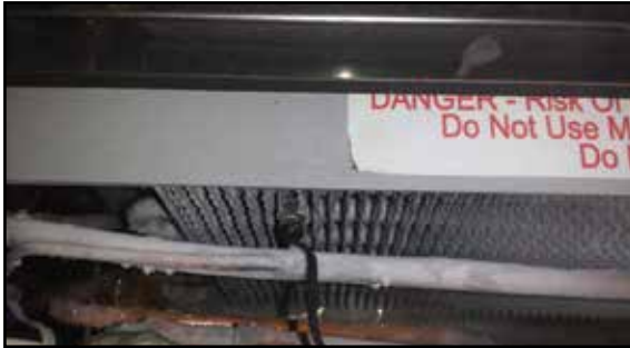
Figure 7-3.1. Evaporator Temperature Probe
