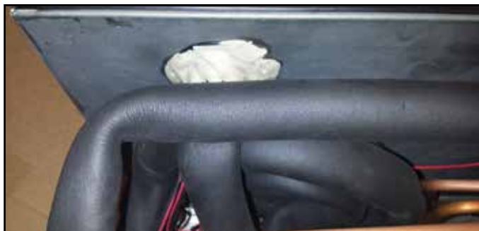
Figure 6-1.1. Sealing Compound (Inside)
