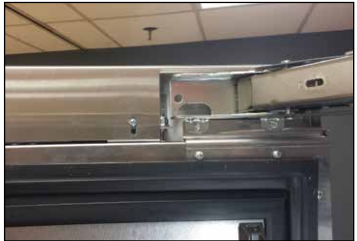
Figure 7-4. Door Magnet (Reed Switch)
