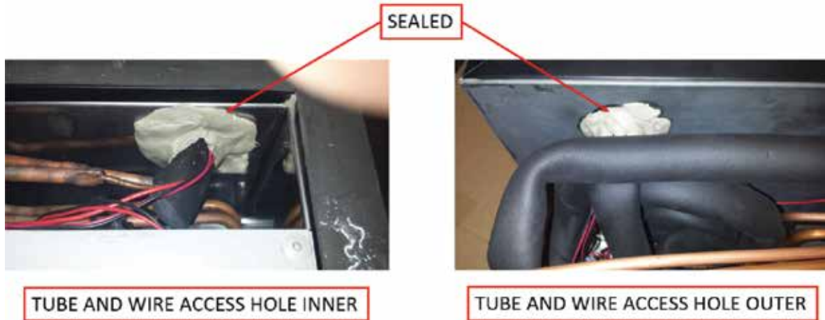
Figure 6-15.9. Seal Access Hole
