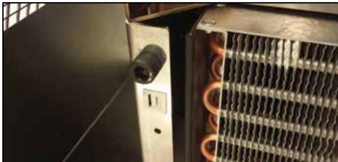
Figure 6-2.2. Lift Bolts
