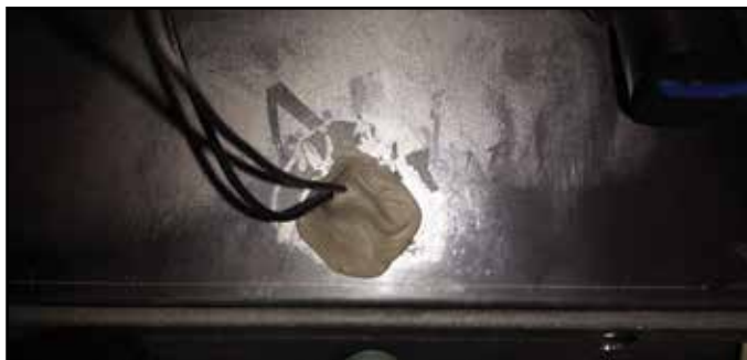
Figure 6-1.3. Sealing Compound - Door Switch (Inside)
