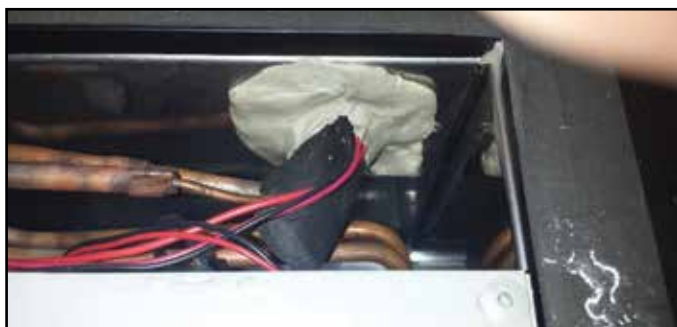
Figure 6-1.2. Sealing Compound (Outside)
