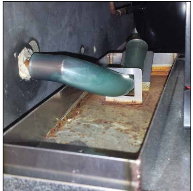
Figure 6-3. Evaporator Condensate Drain
