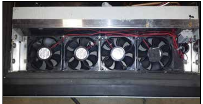
Figure 6-14.1. Evaporator Fan Motor/Fastener
