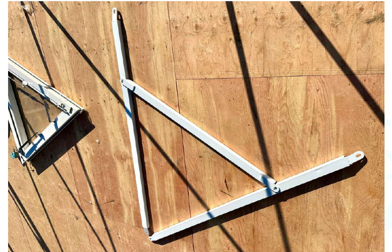
Tubing pieces to add during frame build
