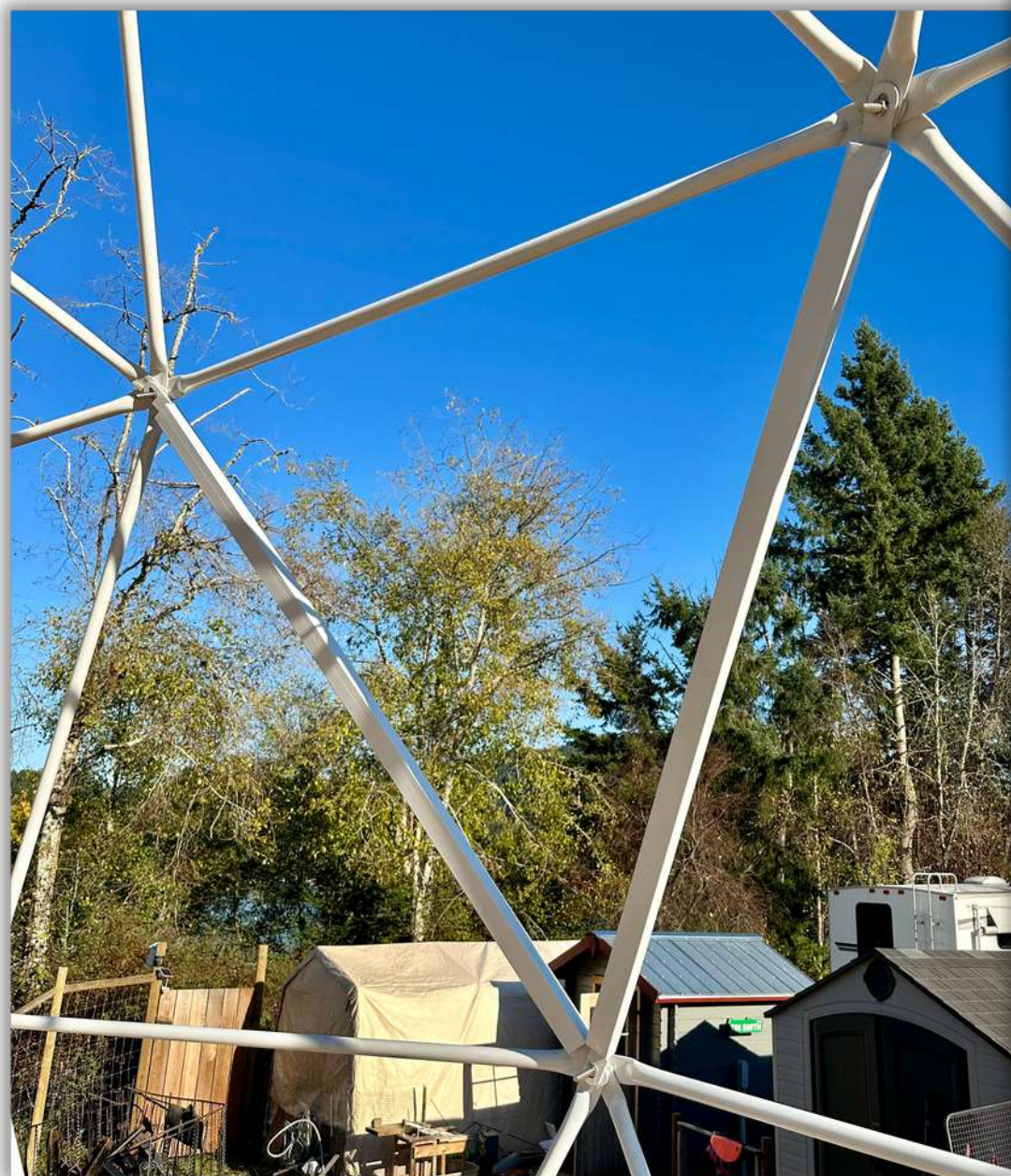
Installed square Tubing frame
