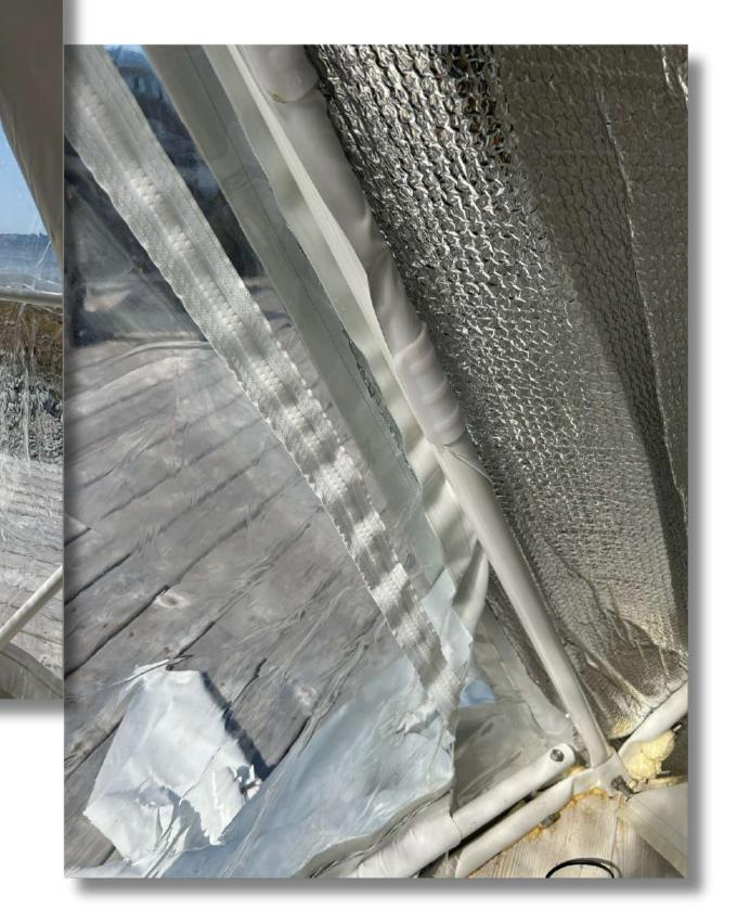
Try to apply some sideways tension on the window when clipping it, or use additional tape to hold it tight.
