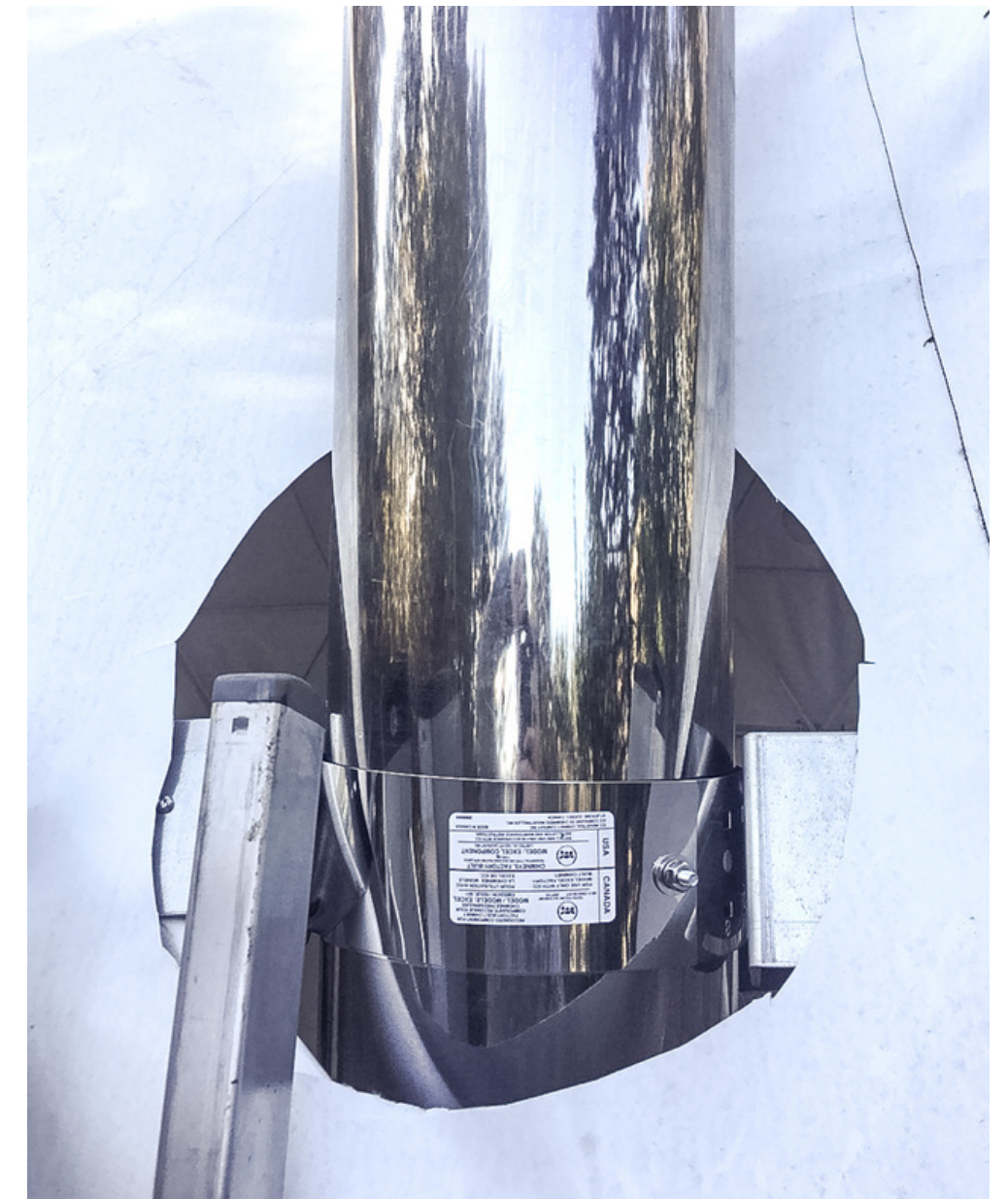
Example shown includes 3rd party chrome chimney support (unnecessary in most cases)
