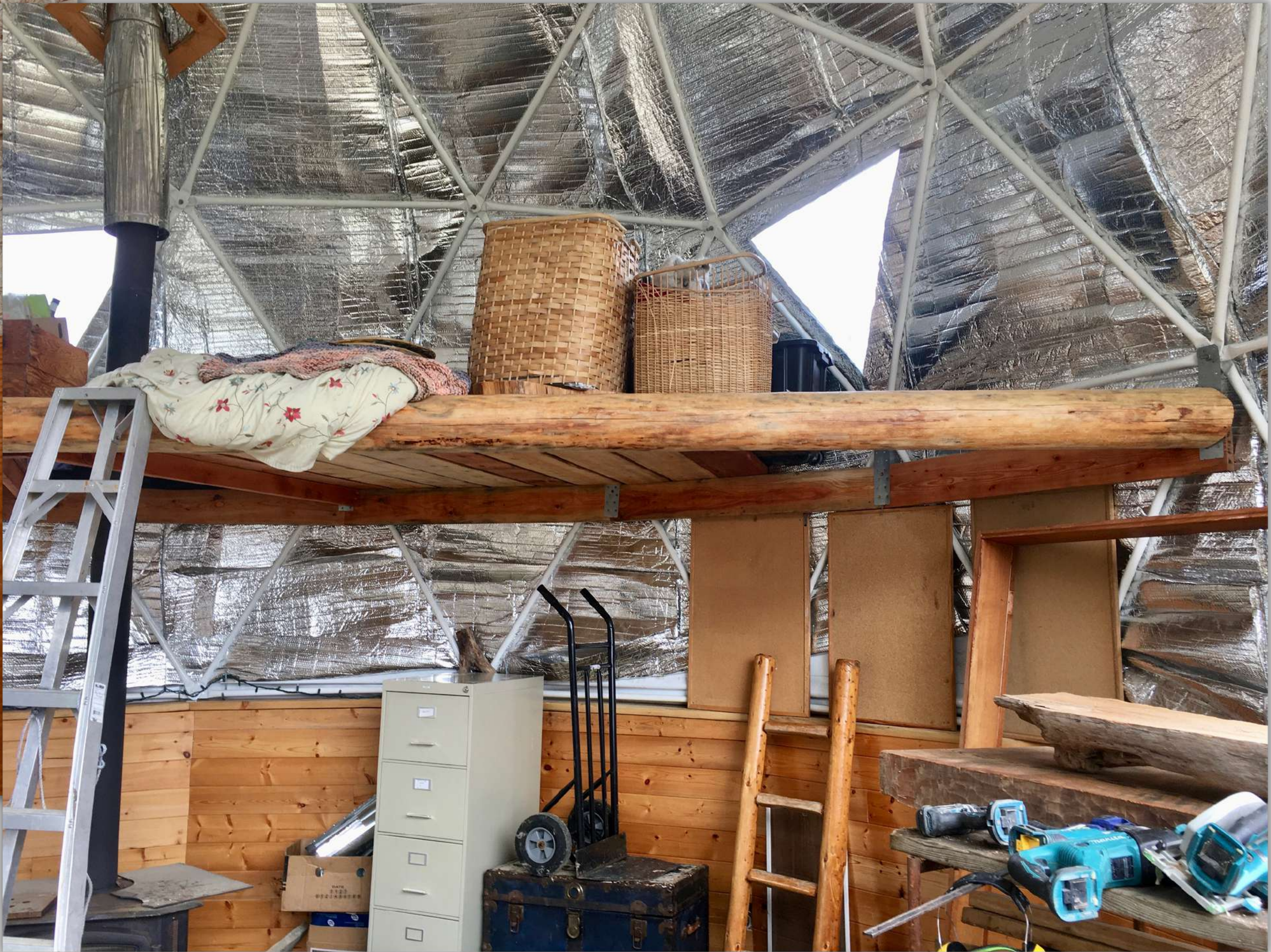
The loft can also be installed after hanging the inner liner.
