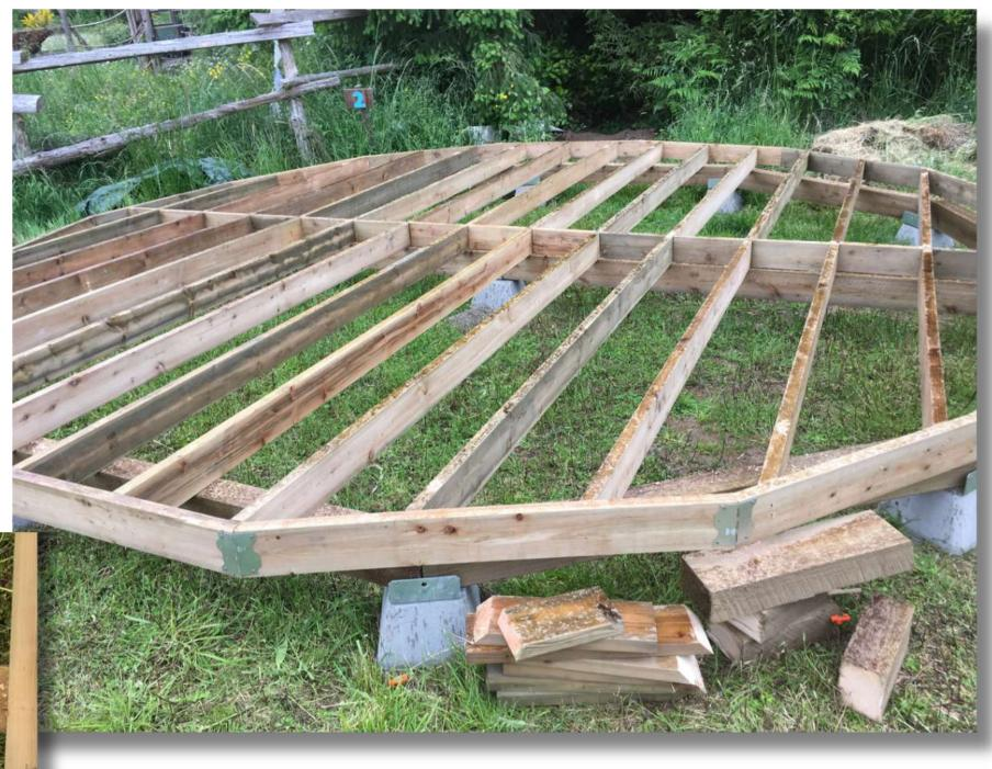
It may make sense to build the joist structure in sections so that it is easier to attach the plywood to the underside.
