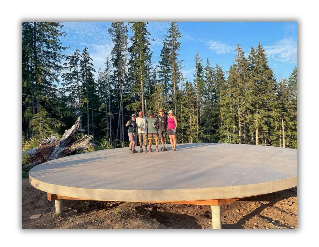
While a round platform can work alright for larger domes (4V or higher frequency), it is not recommended for our most popular 3V domes as the curve would stick out in between the hubs.
