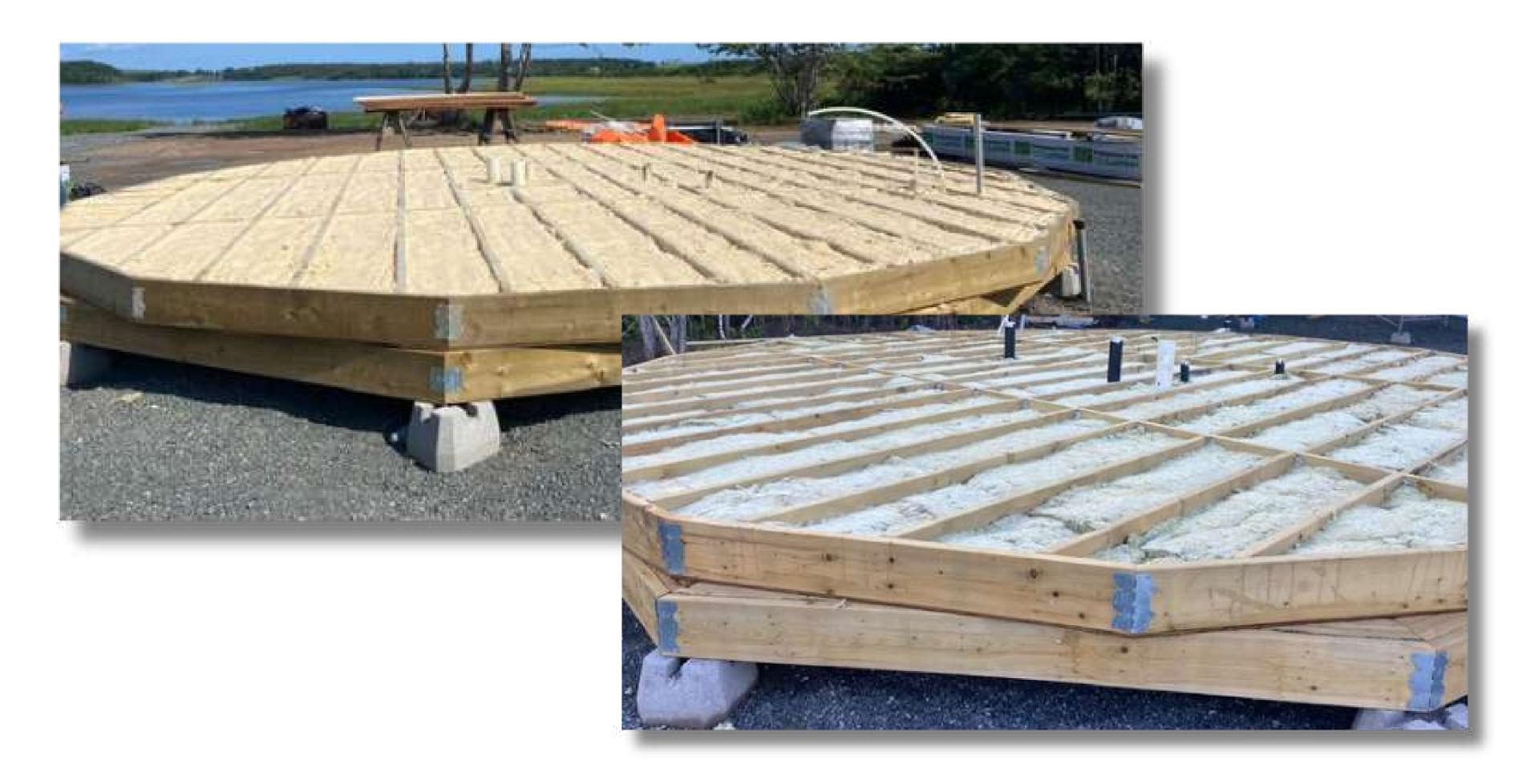
Lay our the subfloor 3/4" plywood on the joists according to the pattern on the plans and screw it down. You may want to use wood filler in the cracks.
