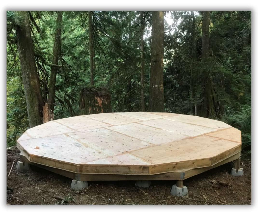
**Tip:** for a low-budget yet beautiful floor, you can use a tiger torch to lightly burn the plywood and bring out the wood grain, and then apply a couple of layers of clear flooring finish to seal it. Please make sure to do this BEFORE you set up your dome so it doesn't light on fire!
