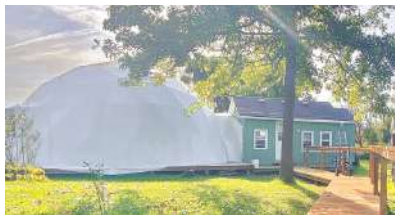
Custom awnings are available for connecting to other domes or buildings
