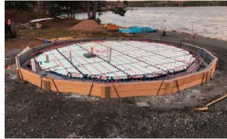
Poured concrete floors (potentially with radiant heat!)
