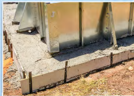
SET WALLS AND BRACING IN PLACE
