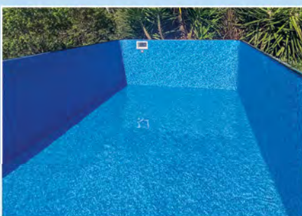
INSTALL LINER AND FILL WITH WATER
