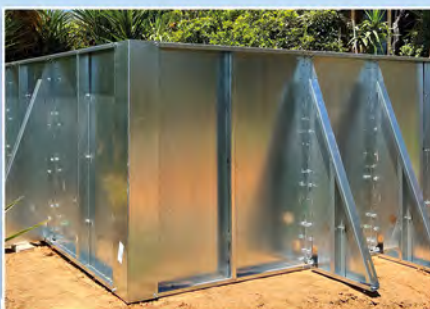
CONSTRUCT WALLS AND BRACING
