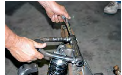
18) Using the other long bolt supplied in the kit, the upper A-arm was installed. This connection also uses the large washers supplied in the kit. The upper bolt is secured with a Nylok locknut.
