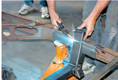
12) After the towers lined up perfectly, they were tack-welded to the frame. All of the measurements were made again to be certain they were correct. When O'Bryant was satisfied, the towers and crossmember were finish-welded to the frame.
