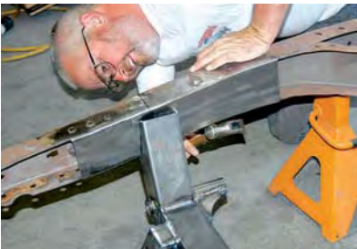
8) The crossmember was installed and it was a tight fit. A few hammer whacks were necessary to get the centerlines to match up.
