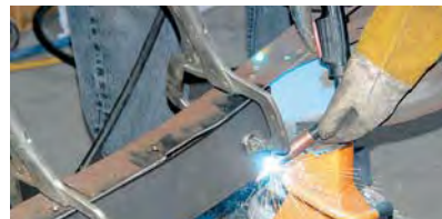
6) O'Bryant decided that it would be better to use a pair of hand clamps to secure the boxing plate before the welding was done. He started by tack-welding the section to the frame at the front and rear.
