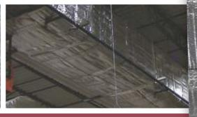
**rFOIL®** BIG-6 Reflective Duct Insulation is a 5/16" layer of polyethylene bubble, bonded to and sandwiched between two radiant barrier sheets. Then, four strips of spacers are pre-attached and run along the full length of the roll. these spacers help provide the necessary airspace to achieve an R-6.0 insulating value.
