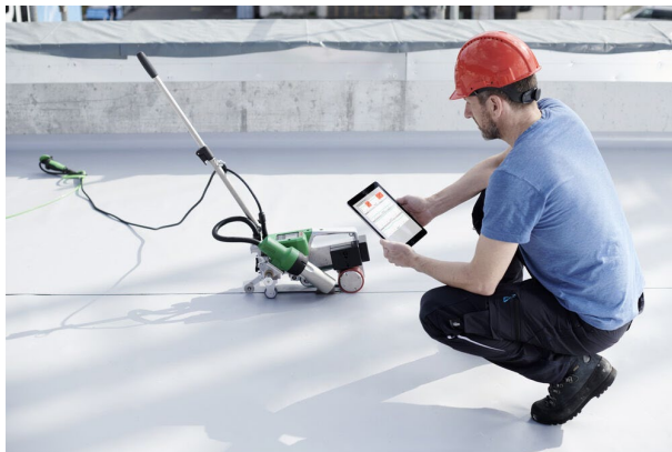
Automatic roof welding machine UNIROOF 700 from Leister: increased safety while welding
